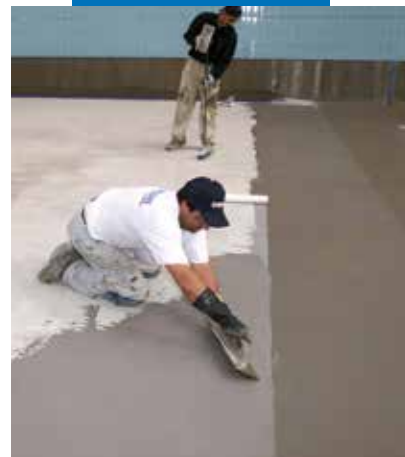
Hydroizolace bazénu Mapelasticem
